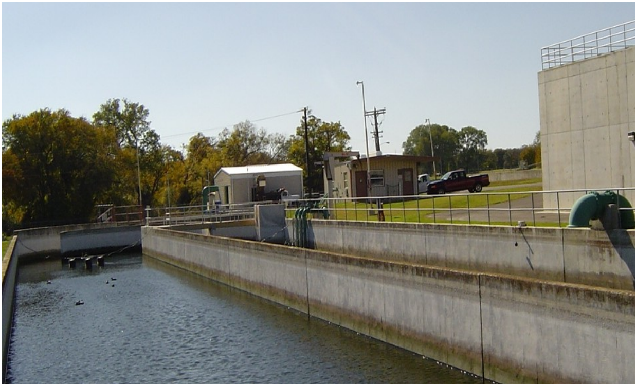
Northeast Wastewater Treatment Plant Equalization basin—A portion of the new Sequencing Batch Reactor (SBR) plan.
