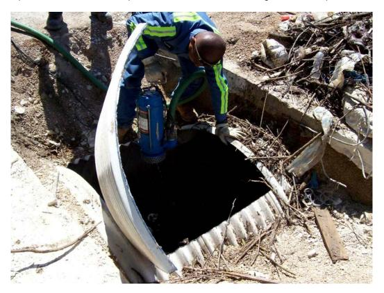
Worker Cutting an Opening in an Underground Corrugated Metal Pipe to Remove Debris Blockage
