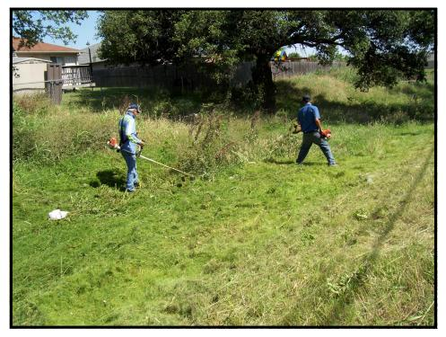
Workers Clearing Vegetation and Debris from Drainage Ditch
