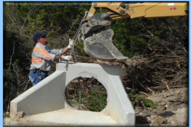
William Colby, Mechanic, along with other employees setting head wall for a concrete culvert
