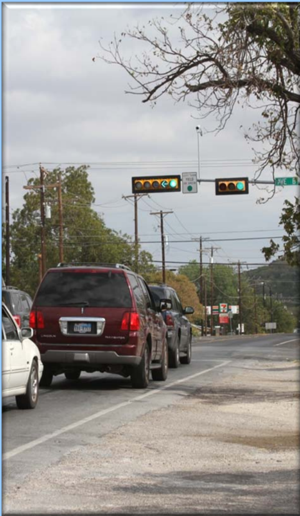
North 1 st Street and West Avenue B received a dedicated left turn lane and signal in 2011
