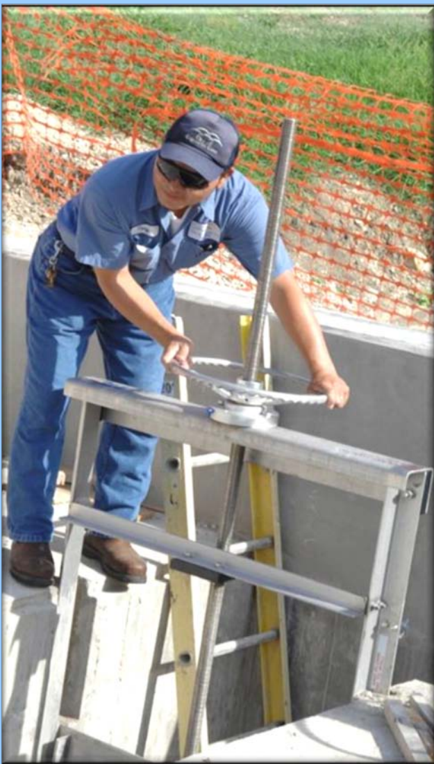
Anthony Castro, Operator II, Northeast Wastewater Treatment Plant
