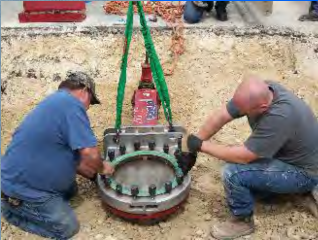
Installing Insta Valves on water main
