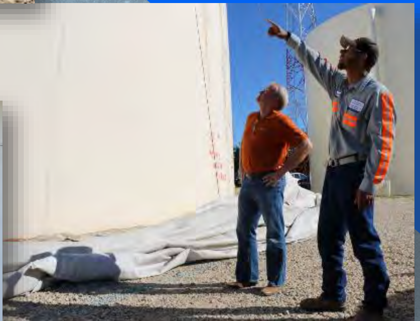
Inspecting water tower renovations
