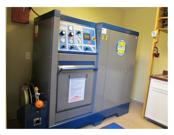
The department received a Bauer Mini Unicus air compressor and air storage system. The air compressor and storage system is used to fill firefighter air packs (Self Contained Breathing Apparatus (SCBA)). The Bauer unit replaced a Bauer Mariner compressor that was about 18 years old. The Bauer Mariner provided almost two decades of service to the department before it was retired.
