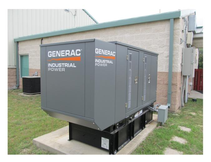
A new emergency back up generator was purchased and installed at Station 3. It replaced a 12 year old generator that had quit working and was unable to be repaired due to lack of the availability of repair parts. The Generator supplies limited power to the Fire Station to ensure that vital systems continue to function when commercial power mains are without power.
