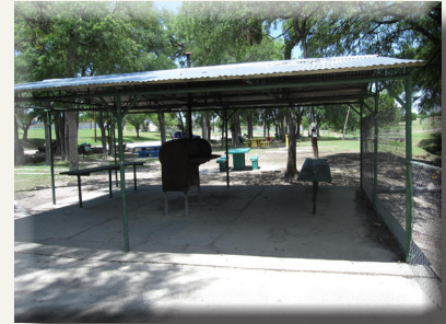
Existing pavilion at City Park.
