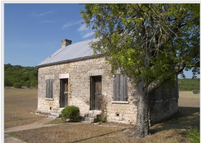
Original post office and stage stop Source: Wikipedia
