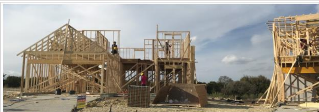
Construction of New Single Family Homes Near Lutheran Church Road
